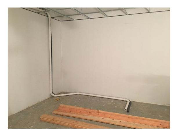
Clean studio power is run in a dedicated conduit. When long runs are required from control room to tracking room and booths, the runs are direct as possible and do not loop around the room. This is accomplished by running the electrical for audio conduit in the ceiling or floor. Run a straight line with short branches as necessary. The audio cabling must run in larger conduit(s) right next to the electrical conduit. This procedure eliminates the loop area in the connected ground wires.
