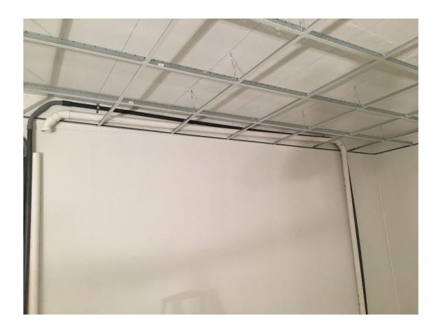
The conduits on the floor will be exposed in the front of the control room and feed the desk/console. This ties them into the system while maintaining a zero-loop area wiring system.
